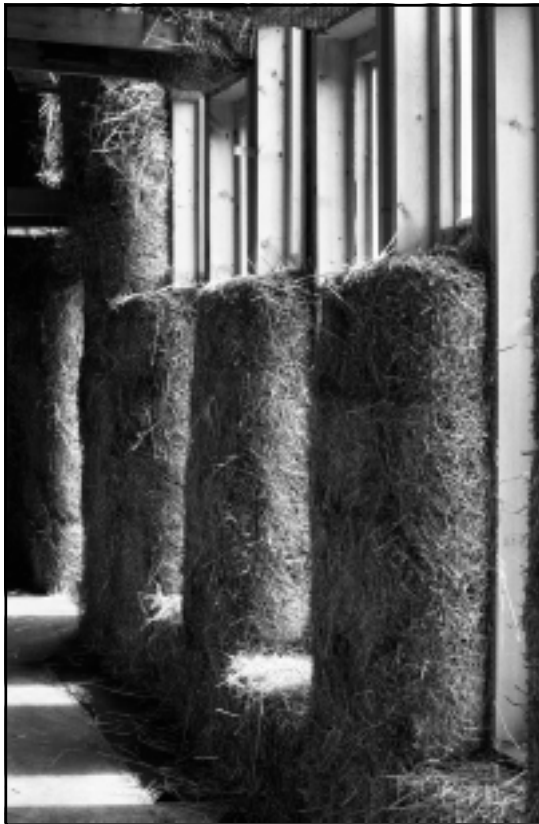
Pre-plaster, south-facing interior straw bale insulated walls.
