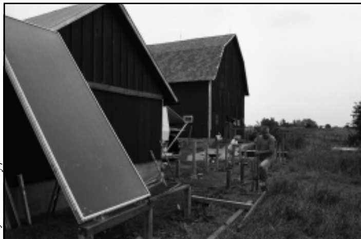
Judy and Phil Welty setting posts for solar collectors.
