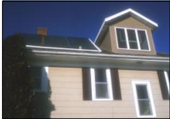
Solar thermal system for domestic hot water, alongside dormer with low-E windows.
