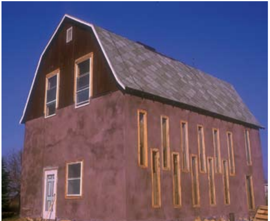
An old granary and corncrib was reconstructed as a straw-bale-insulated greenhouse with the help of neighbors, friends, and installation workshops by the Midwest Renewable Energy Association.
